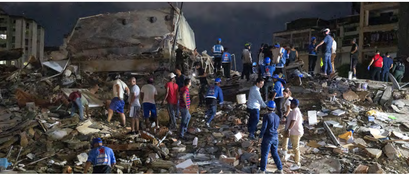
IMAGES of completely flattened buildings continue to emerge as the death toll is expected to rise significantly over the coming days.
